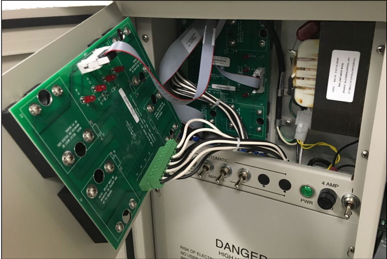
Figure 22 Completed Install of 50-Amp Pump Relay Assembly (198633D)
