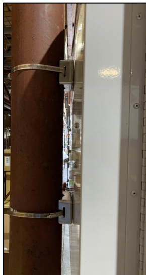
Top and bottom bands installed.
