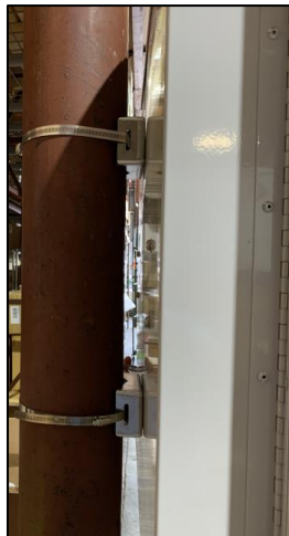
Top and bottom bands installed.
