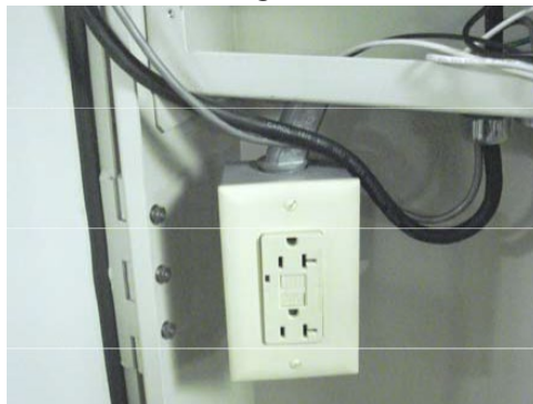
Figure 15. Outlet Box Installation
