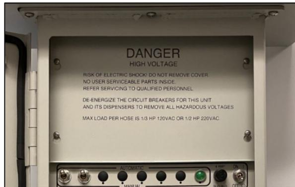
Figure 30 Replacing the Upper Pedestal Cover Plate
